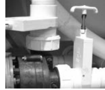
Slice Valve and Pump Union
